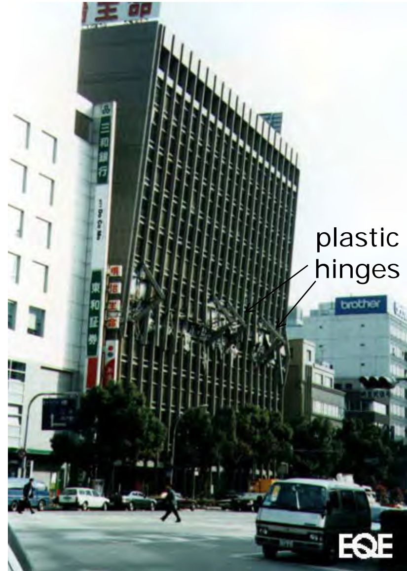
Mid-story collapse, 1995 Kobe earthquake (EQE Summary Rep., 1995)
